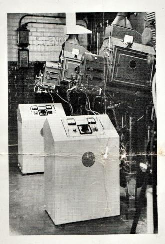
The alternative cable entries enable the rectifier to be placed at right-angles to the lamp if there is insufficient room in the projection box between the rear of the lamp and the back wall. If it is desired to use remote control the instrument panel can be removed readily and fitted in a convenient position at the lamp or front wall while the rectifier itself is installed in a separate rectifier room.
