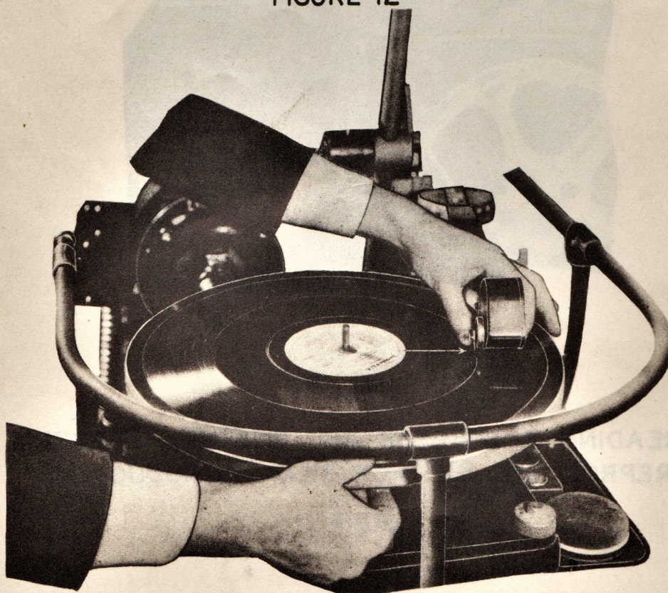
METHOD OF SETTING RECORD AT STARTING POINT ON WESTERN ELECTRIC REPRODUCER SET
