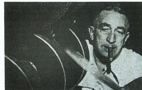
Harry Squire, Cinerama photographer, filmed many of the most dramatic sequences of "This is Cinerama." He is shown threading the triple magazines of the three-lensed camera which captures virtually the entire range of human vision on its multiple film strips.
