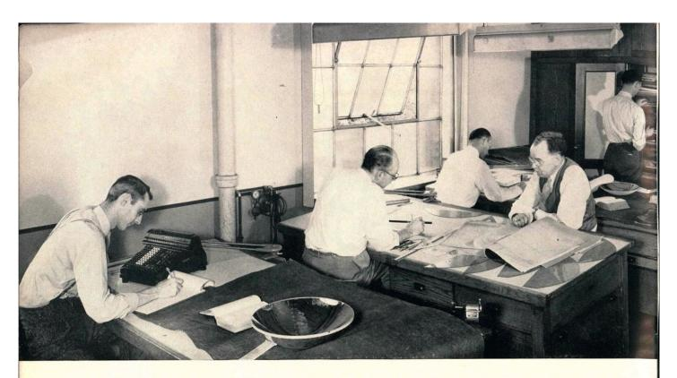
The design of an elliptical reflector requires a staff of skilled technicians to compute the exacting physical and optical requirements necessary to pick up the light from the positive arc crater and focus light accurately at the film aperture.
