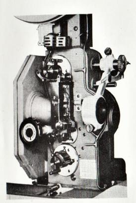
The Gaumont-Kalee '21' model (illustrated at right with cover removed) is a totally-enclosed mechanism incorporating force feed lubrication, double aperture mask plate with twin threading lamps, single blade shutter running at twice normal speed, giving approximately 20% increase in light efficiency with less flicker and improved definition, electrically operated change-over device and many other refinements.
