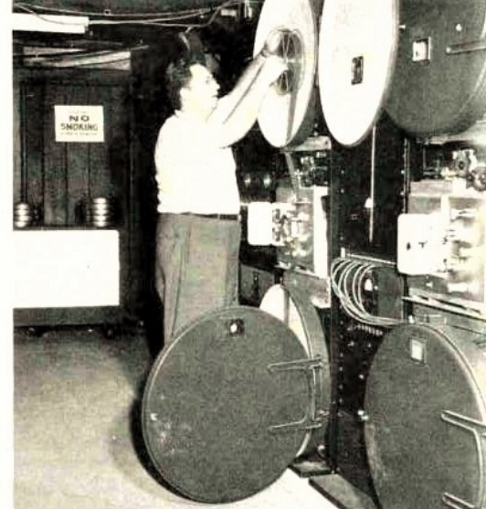
The Cinerama "sound head" which picks up the sound from the seven iron oxide tracks, carried on a single strip of 35 mm film, and feeds it to the loudspeakers in the theater.
