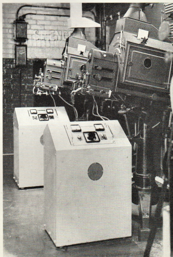
Single-phase cinema arc rectifier installed in the A.B.C. Regal Cinema, Caversham, Reading.
