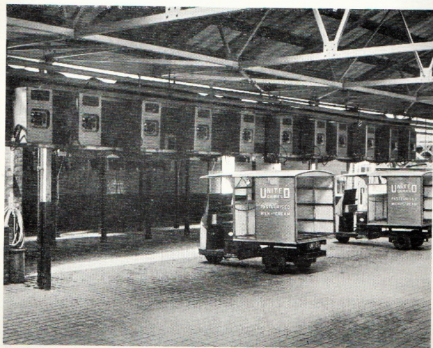
Fig. 58.—Typical installation of vehicle chargers at the Tulsa Hill Depot of United Dairies. (by courtesy of Mickleover Transport Ltd.).
